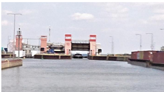
Sharnebrucke Ship-Lift capable of handling 3,000ton barges
